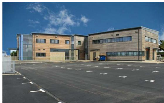
The building consisted of the construction of a steel frame extension, enveloped with a mixture of facing blockwork, cedar cladding and curtain walling.
