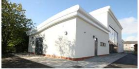
A new-build sports and dining hall, including commercial kitchen and storage, plant room, toilets and changing room. Constructed in steel frame, with a standing seam roof, a curtain walling with insulated external rendered finish.
