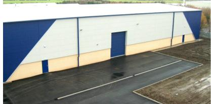
This Design & Build project consisted of the construction of a structural steel portal frame supported on a reinforced concrete ring beam enveloped with a mixture of facing brickwork and composite/build-up cladding.
