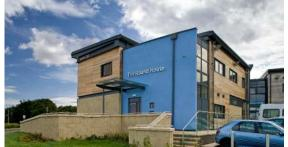
The building consisted of the construction of a steel frame extension, enveloped with a mixture of facing blockwork, cedar cladding and curtain walling.
